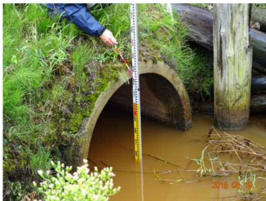
横断管の通水状況 管径φ1200mm
